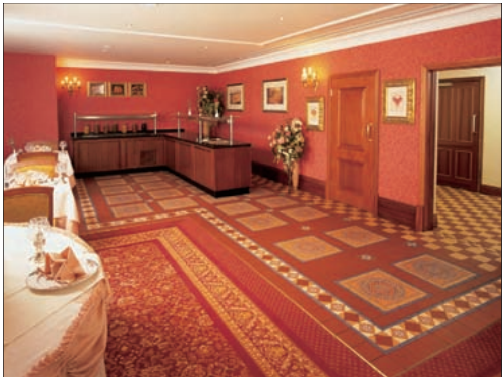
Blue decorated Disraeli centrepiece panels in a frame of 149 x 75 x 50mm buff trapezium tiles and 151 x 24mm blue rectangles, with individual blue/white Liverpool tiles and a modified Scott border.
